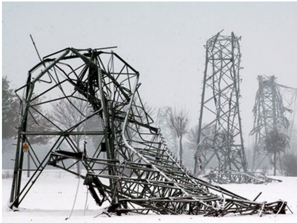
Fig. 10. Collapsed towers in Slovenia, February 2014
